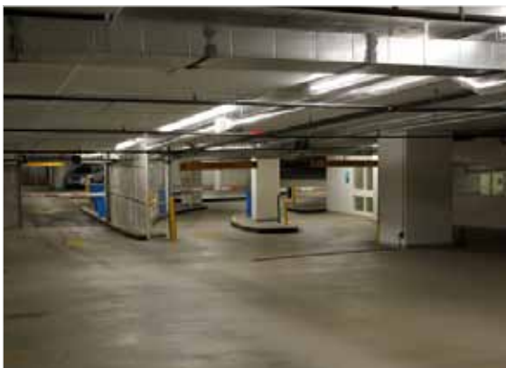
Kryton's concrete waterproofing system was used to protect all below grade areas.
